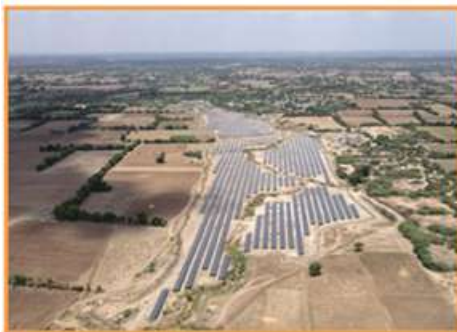
6MW Ground Mounted Solar PV Plant at village Sujjanpura
