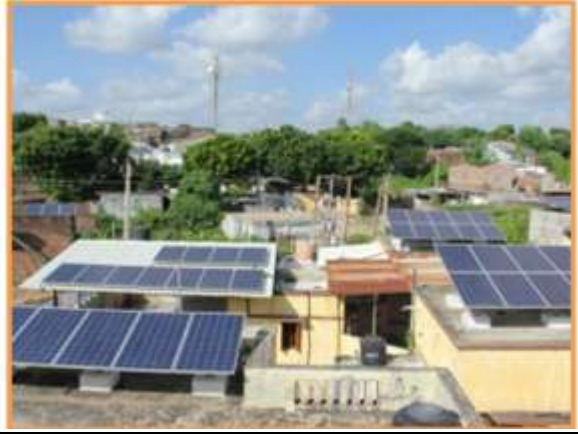
100kW Roof Top Systems on Government Buildings at Modhera
