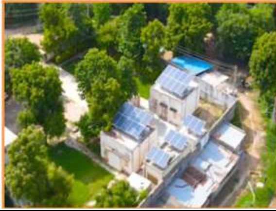
100kW Roof Top Systems on Government Buildings at Modhera
